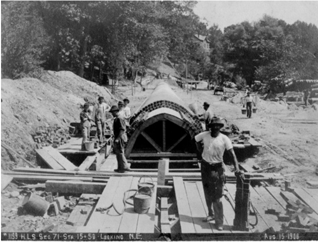
The 9-foot-diameter sewer line being installed in Bussey Brook Meadow in August 1900.
